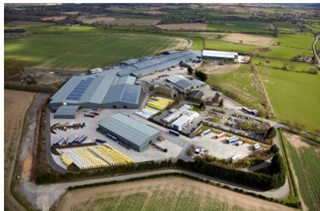
Kingspan Insulation's Pembridge site has recently been awarded a World Class Operation Management Gold award.
